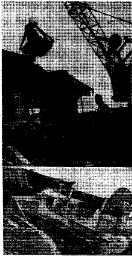
(TOP) Edward Berryman, industrial equipment operator foreman, watches 20 ton crane demolish ice house. (BOT.) Wendell Timm tears into structure with his bulldozer. (Photos by Jack Strood.)
